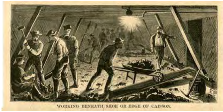
Working beneath shoe or edge of caisson.
