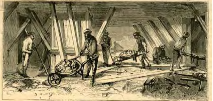
SENDING UP DÉBRIS THROUGH THE WATER SHAFT.
