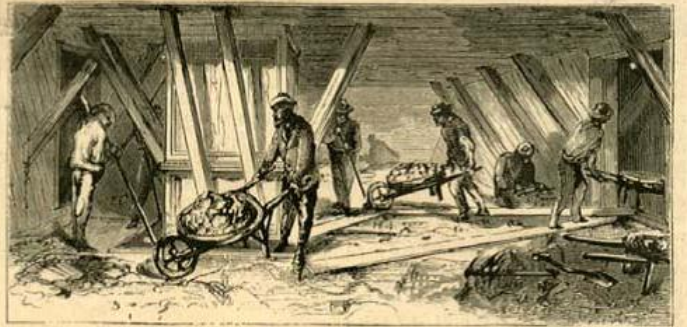
SENDING UP DÉBRIS THROUGH THE WATER SHAFT.
