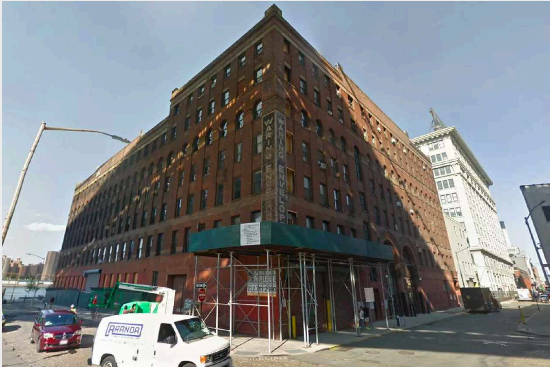
Waring Envelope sign still visible on the corner of the building
