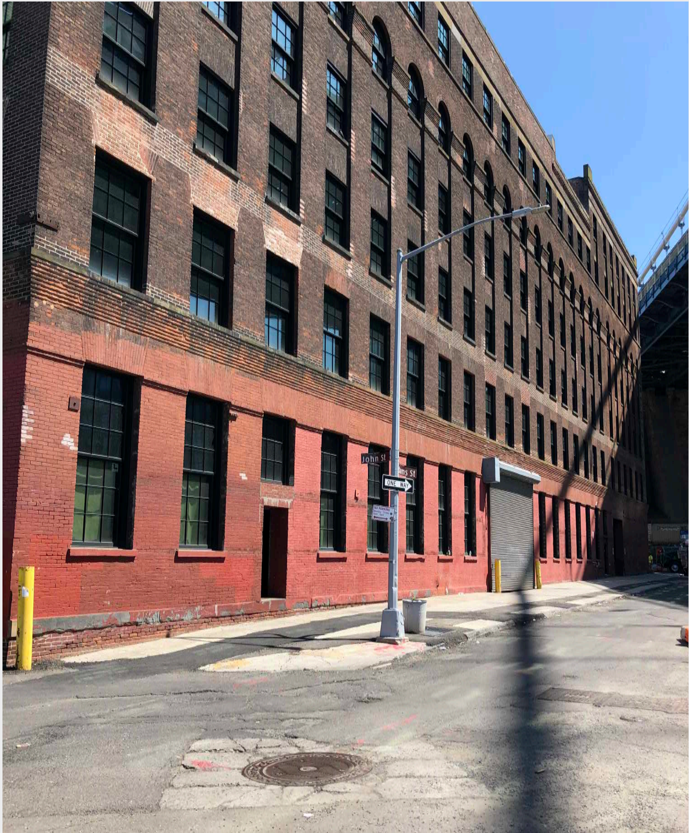
Facade on Adams Street, the entrance side.
